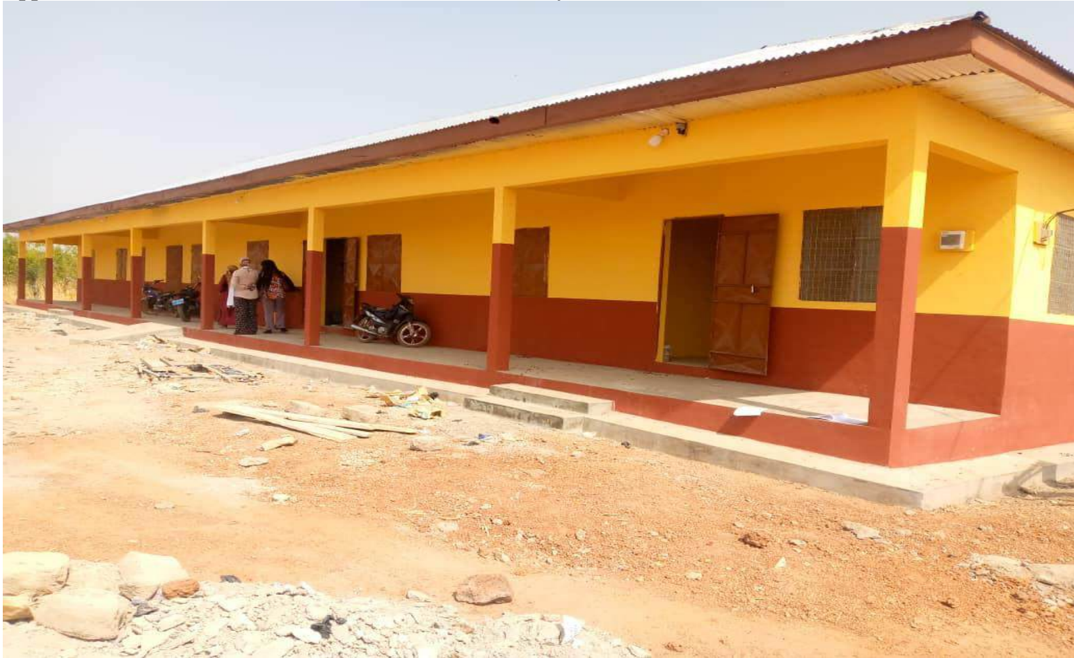
Appendix 7. Picture of 3-unit classroom block at Kukuonayili
